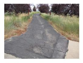
This component provides funding to do a 2-inch mill edge and overlay. Poor conditions observed. This is recommended every 30 years.
