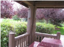
The 4 - 2 foot diameter Log Posts 10' high are in good condition with some cracking. This component provides funding to repair or replace as needed.
