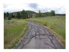
This component provides funding to do a crack fill on the asphalt in the community. At a minimum, this needs to be done every 6 years. The trail system within the community is in need of some major repairs.
