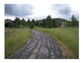
This component provides funding to do a slurry seal on the asphalt. Poor conditions observed. At a minimum, this needs to be done every 6 years.
