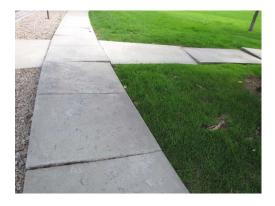
This component provides funding for the 4600 SQ FT of concrete within the community to be repaired or replaced as needed. The sidewalks, and pads in the community are in fair condition with some cracking, settling, and surface pealing.
